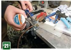
We were not satisfied with the crimp alone, so out came the soldering iron and crocodile clips for a much more substantial and water-resistant connection. The entire charging circuit relies on two of these terminals so it needs to be a very good connection.
